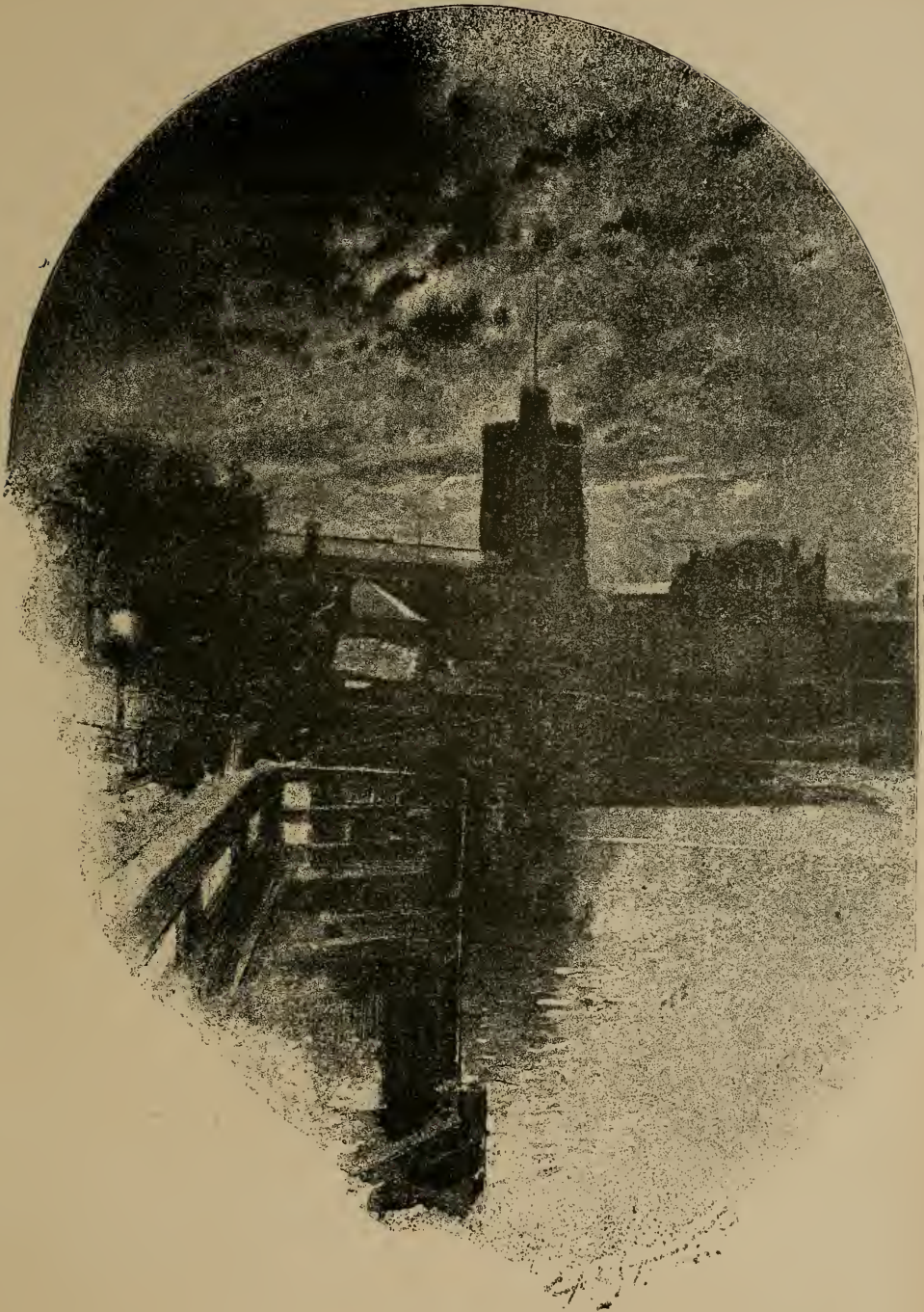
OLD PUTNEY BRIDGE.
